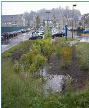
Villanova University stormwater bio-infiltration traffic island BMP
